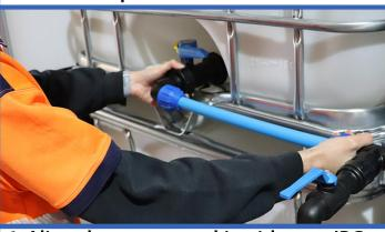
6. Align the connector kit with your IBCs valves and thread the IBC connectors on.
