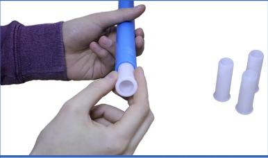
2. Insert PL pipe liners into both ends of each section of MDPE pipe.
