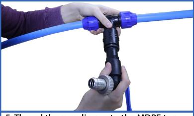
5. Thread the coupling onto the MDPE tee piece until firmly secured.
