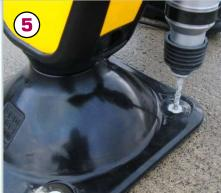
Using the product base (with nylon spacers fitted) as a jig, drill 10mm diameter holes to a depth of approximately 5-10mm, to mark hole centres.
