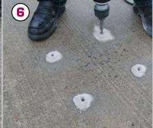
Remove bollard and continue to drill out 4 holes a total of 80 - 90mm depth using a 16 mm masonry drill bit. Remove all loose debris from the holes.
