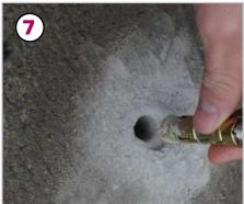
Screw the 100mm button head screws into the Position product centering the four holes. base of the anchor. Ease into the holes until the faces oncoming traffic. Place the large washers top of the anchor is flush with ground level. Tap over the button head screws and place through lightly with a hammer if necessary.
