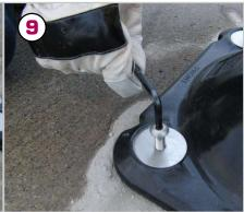
The fixing screws should drop down until they anchor shields so the thread end is just past the Remember to make sure the front of the bollard reach the threaded part of the shield. Make sure all four bolts are engaged in the shield thread by 2 or three turns then proceed to tighten all four bolts to torque setting 27.
