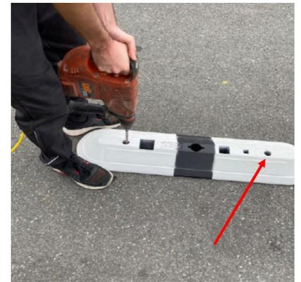
Drill two guide holes using base as a template.
