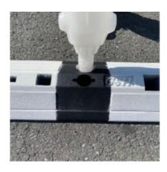
7. Push the CLS bollard stem into bayonet insert
