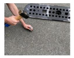
4. Use a hammer to place the two plugs into the holes
