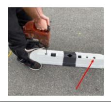
3. Drill two guide holes using base as a template
