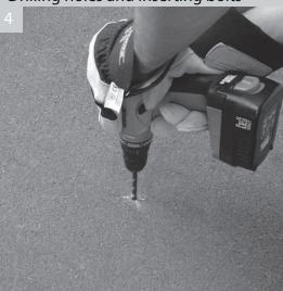
to a depth of 100mm to accommodate the bolt length, remove debris from holes
