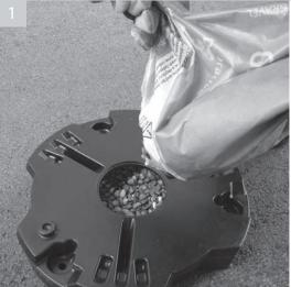
Remove cap and Pour gravel into the cartridge equally disperse gavel across the ballast cartridge fill to 30mm from top, replace cap
