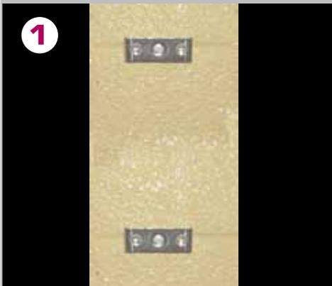
Screw the bracket and spacer into the wall holes, repeat for second bracket.
