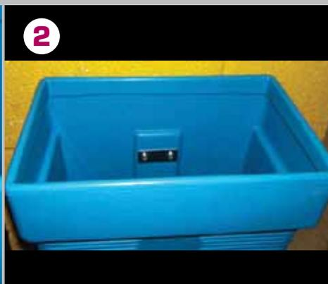
Position up the metal plate and screw in the machine screws lightly repeat for both brackets.
