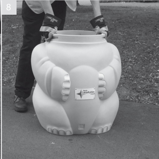
Replace bin locating over ground holes
