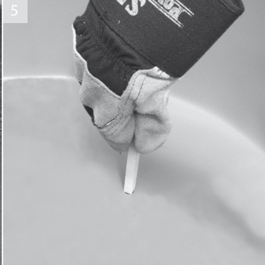
Position the body in the correct location and orientation. Mark through the holes in the base to the ground below
