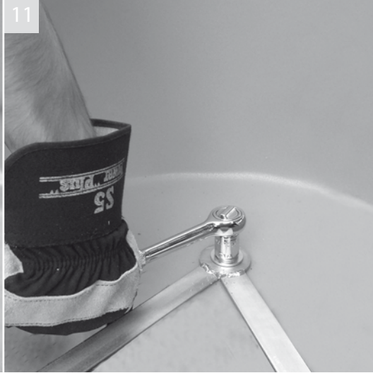
Use a spanner or socket to tighten the bolts. Tighten to 22.0Nm torque for concrete.
