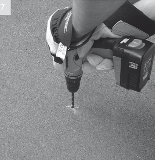
Drill 12mm holes in the four marked positions to a depth of 70mm to accommodate the full length of the bolts. Clear debris from holes
