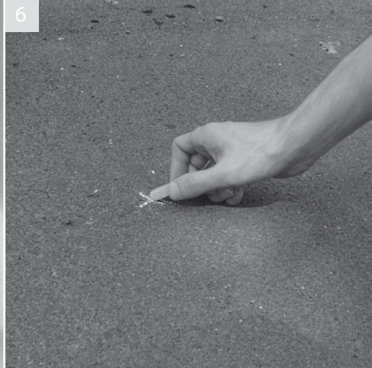
Remove bin body and clearly mark the ground below in the three bolt locations
