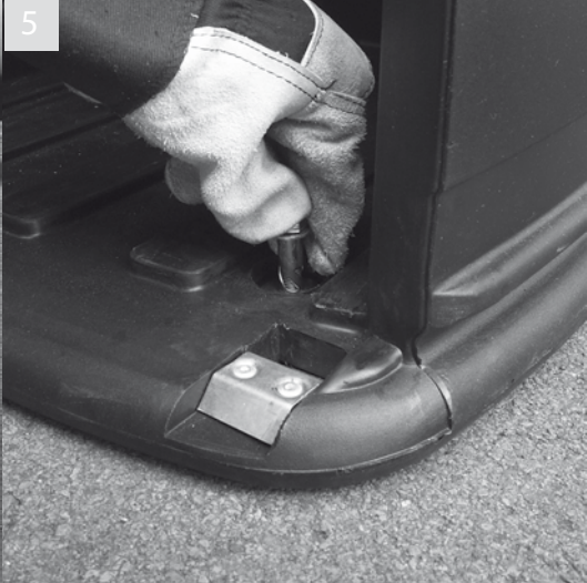
5 Re-position the bin over the drilled holes. Add washers to bolts and push through moulded holes in base into drilled ground holes
