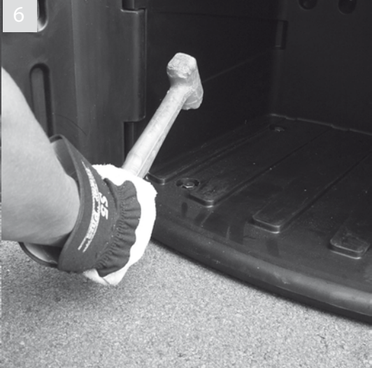
6 Using a mallet drive the bolts home
