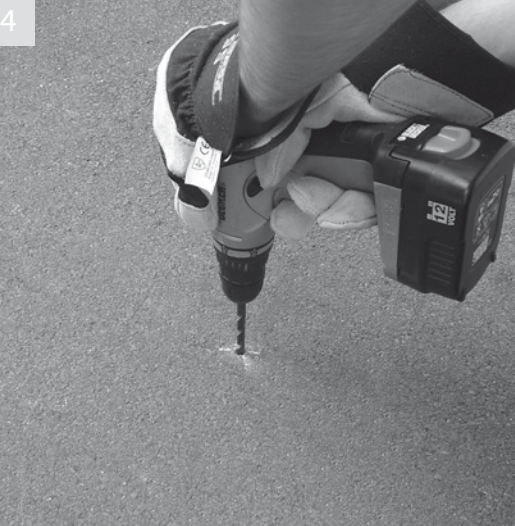
4 Drill 12mm holes in the four marked positions to a depth of 100mm to accommodate the bolt length. Remove debris from holes
