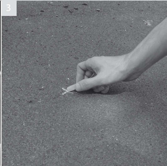
Remove ballast cartridge and clearly mark the ground in the three hole positions with a cross
