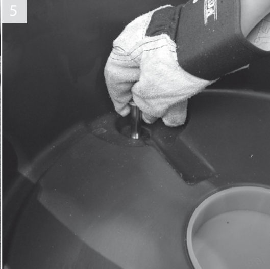
Re-position the base over the drilled holes. Add washers to bolts and push through moulded holes in base locating into drilled ground holes
