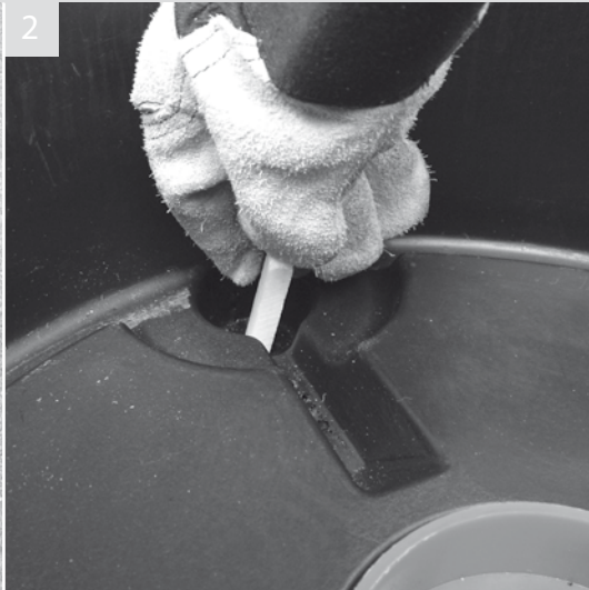
Using chalk, mark the position through the three holes onto the ground below
