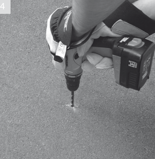
Drill 12mm holes in the three marked positions to a depth of 100mm to accommodate the bolt length, remove debris from holes
