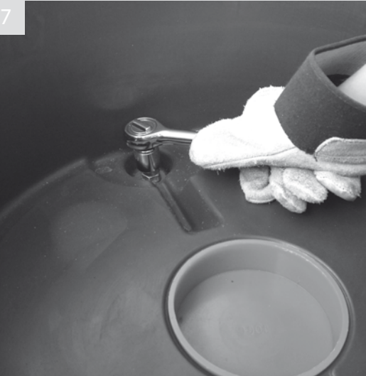
Use a spanner or socket to tighten the bolts
