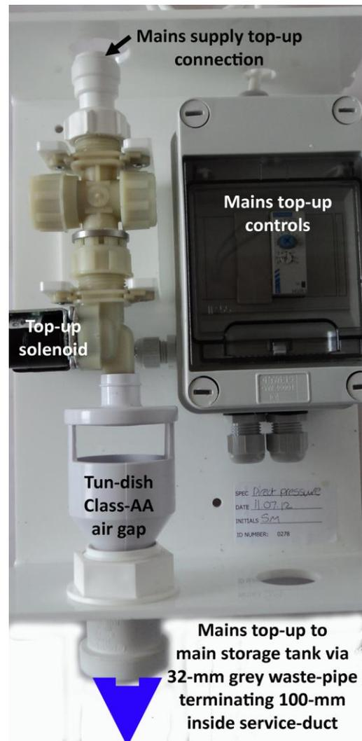
⇒ **Electrics:** Connect the 13-amp supply, pump power cable and top-up cable as shown below:
